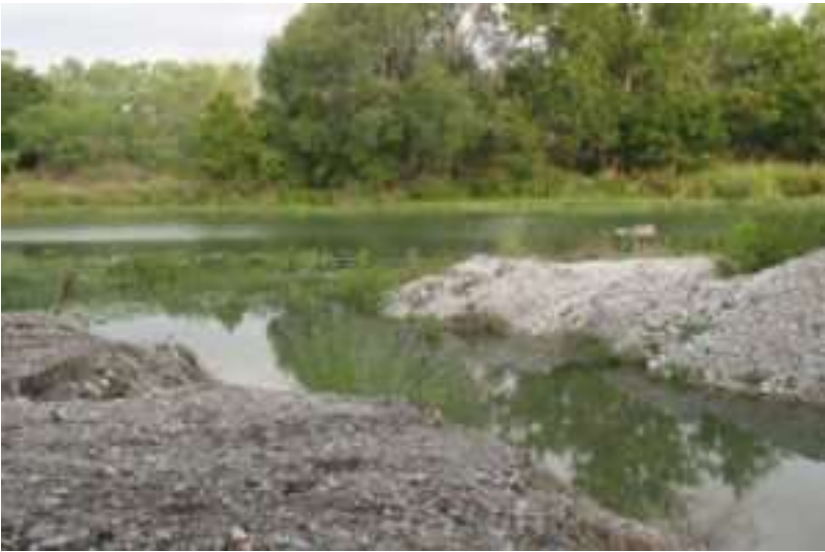
The diversion point of the ditch.
